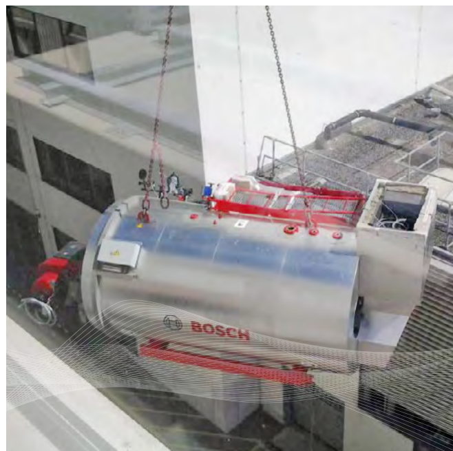
| Placing the boiler in the boiler house
