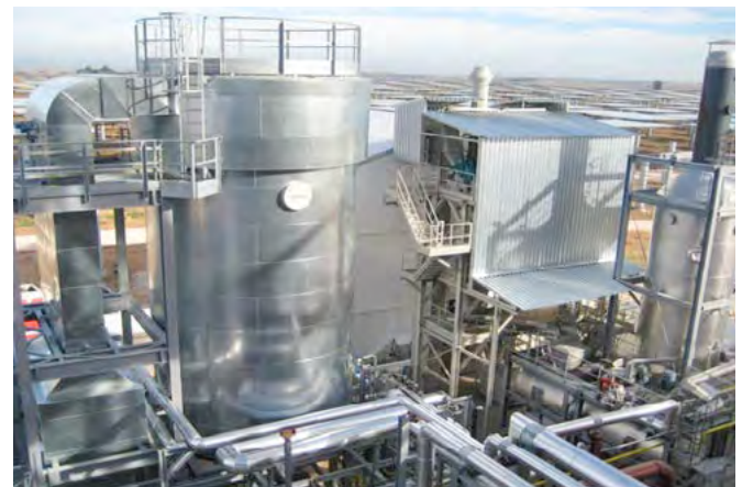
| Molten salt heater system for initial melting of the salt but also as back-up heater up to 560°C flow for thermal solar systems
