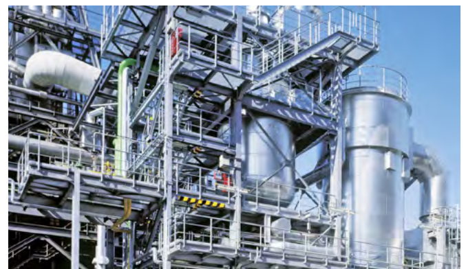
| A bottom-fired heater 26 MW for PET in NL
