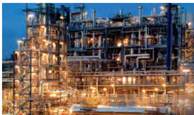
| Two boiler plants 9.5 MW for melamine in DE
