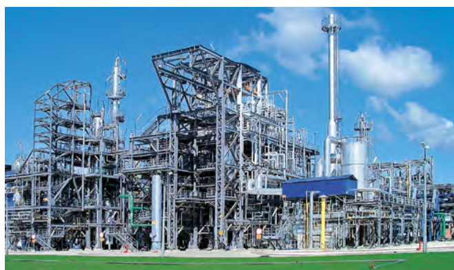
| A boiler plant 8 MW for melamine in PL
