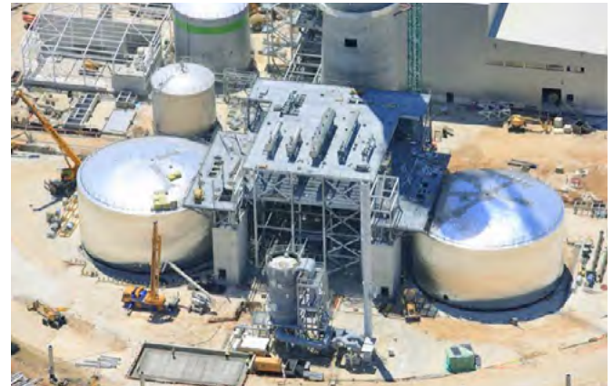
| Molten salt heater system for initial melting of the salt but also as back-up heater up to 560°C flow for thermal solar systems
